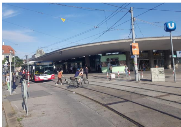
Abbildung 33: Station Hietzing, Busstation © Team Focus
